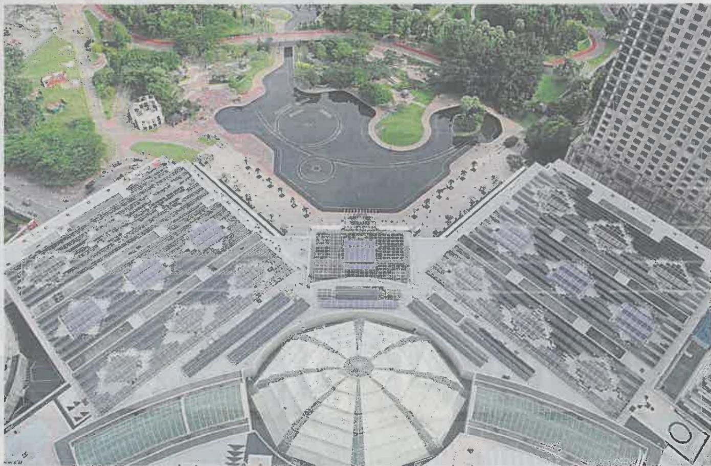
**A bright harvest:** The roof of Suria KLCC no longer sits idle. The 685kWp photovoltaic system installed there can supply 30% of the mall's energy needs or power 250 typical Malaysian households for a month. It saves emission of 360 tonnes of carbon dioxide annually. — Suria KLCC
